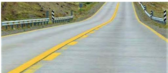
Obajana-Kabba Road (Kogi state) 44 km
